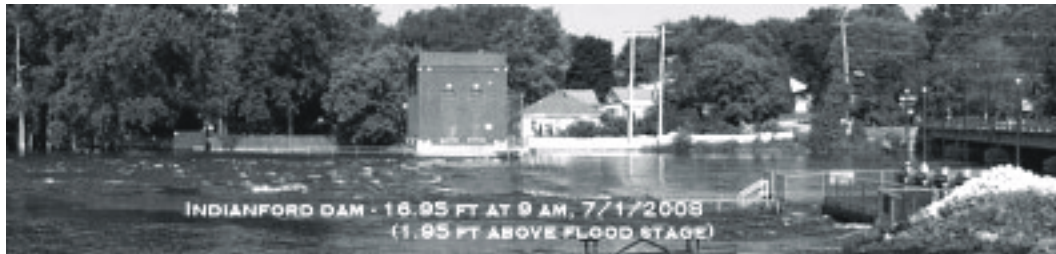
At the peak of the "Flood of 2008," water was flowing across the Indianford dam at rates of more than one million gallons of water per minute.
